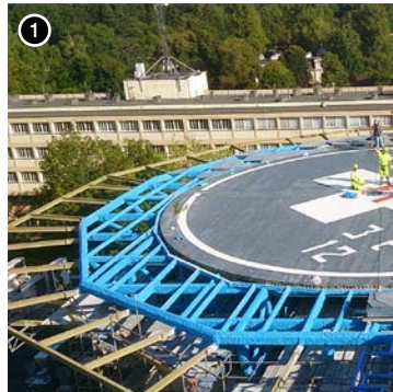
1. Heliport - Olsztyn Hospital, Poland.
