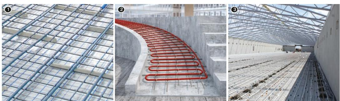
KAN-therm NET is a system of heating pipes mounting on various types of surfaces (on thermal insulation, on the ground, on concrete base). The design of surface heater (or cooler) may differ depending on the applied thermal insulation (or lack thereof) and on the type and thickness of layers over the pipes.
