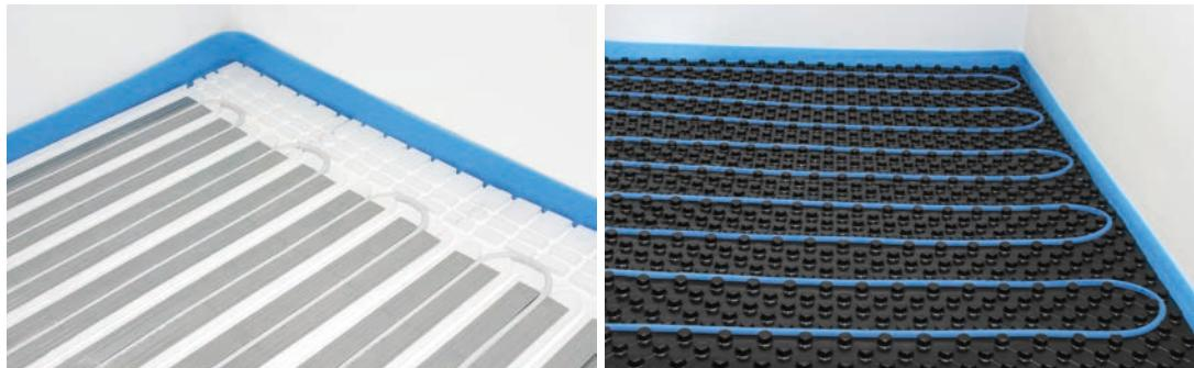
All heating plate contact points with vertical building partitions should be separated by a perimeter dilatation (spacing of at least 5 mm must be maintained). Dilatation should also be performed along the entire length of the doorway thresholds.
