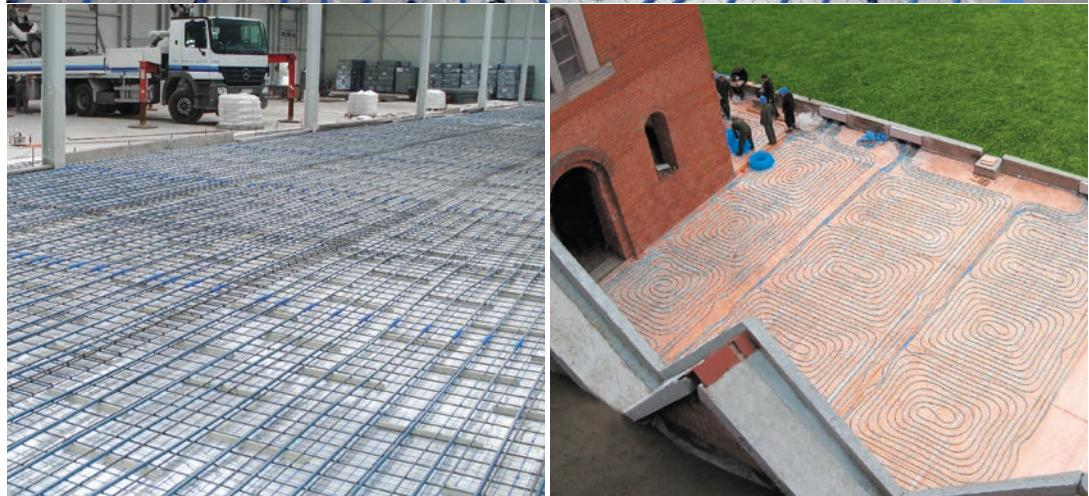
**Fig. 5.** Heating installation of outdoor patio employing KAN-therm system PE-RT pipes.
